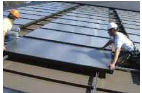
Solar panel installation
